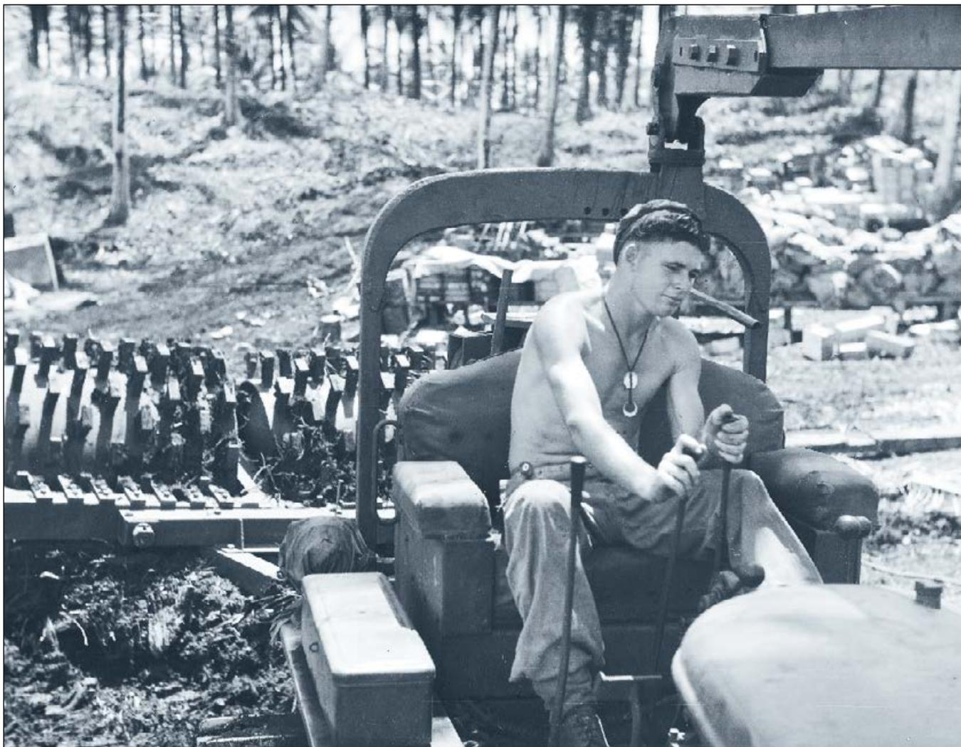
Lance Corporal CF Harvey, 2/3rd Railway Construction Company, Royal Australian Engineers, uses a heavy tractor to haul a roller along a section of new road between an airstrip and camp area at Palmalmal Plantation, New Britain. Development of the 5th Division's base and infrastructure to support the planned land campaign began as soon as engineers and equipment were landed during November 1944. (AWM 077405)
