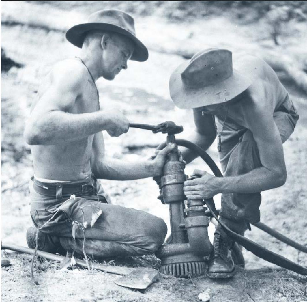
Sapper William Tester (left) and Sapper D'Arcy of the 13th Field Company, Royal Australian Engineers, connect up a compressed air sump pump used for pile driving, during the building of a new bridge across a creek in the Jacquot Bay area in December 1944. Dozens of bridges were needed to traverse the many creeks and streams in the area. (AWM 077662)
