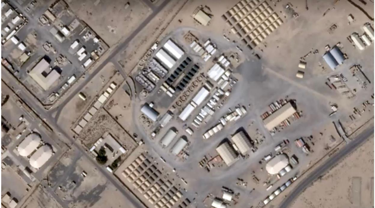
Damage to buildings on a Kuwaiti military base which hosts American troops. Planet Labs PBC
