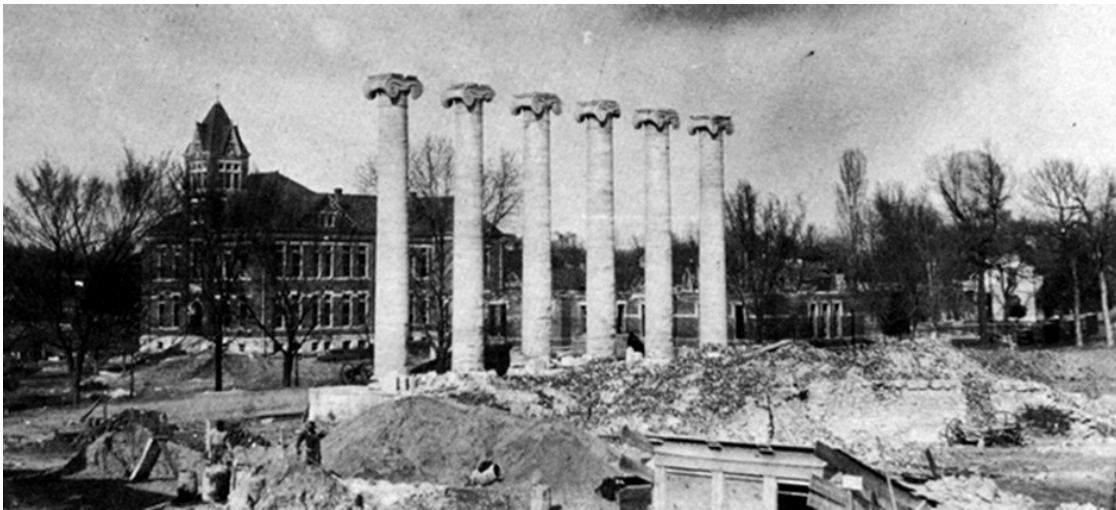
Only the Columns remained after the fire in 1892. In August 1893, the Board of Curators voted to remove the Columns, considering them not only unsafe but also unsightly. However, supporters of the Columns rallied to their defense, and after inspection showed the foundations were safe, the board voted in December 1893 to retain them. Photo courtesy University Archives, Bulletin, 11/22/1971.
