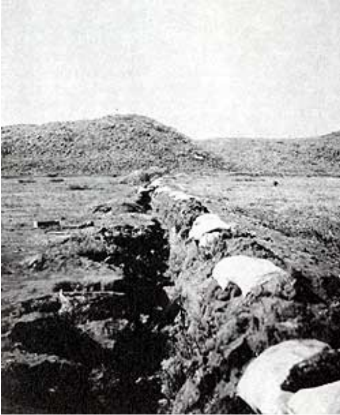
The main Boer trench from which the Highland Brigade was decimated.
