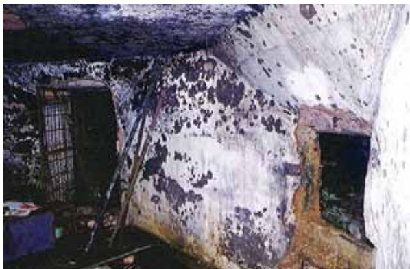
Figures 8a & 8b: The area around the middle firing loop. The left firing loop was converted to an entry. Note the slot at the right side of firing loop and the damaged stand.
