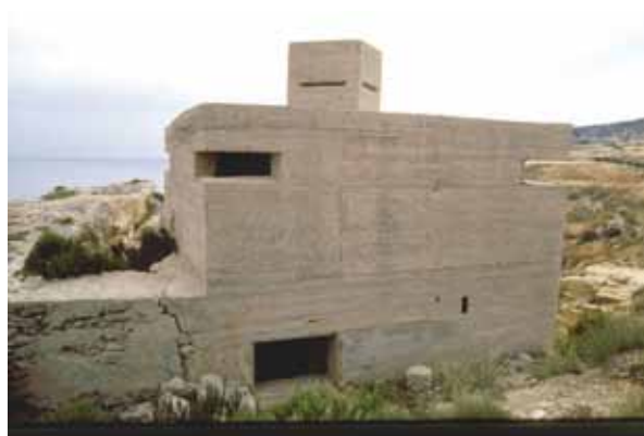
Figure 6: Another pillbox on Marfa Ridge but dating from WW2. It is likely that its concrete sides were painted with a camouflage pattern to resemble that in photo GDL 5. The large opening at its base may be an emergency exit.
