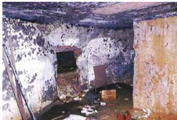
Figures 8a & 8b: The area around the middle firing loop. The left firing loop was converted to an entry. Note the slot at the right side of firing loop and the damaged stand.
