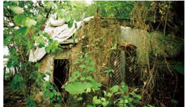
Figure 5: The entry converted from a fire loop. The original entry still can be seen on the right side of the photo.
