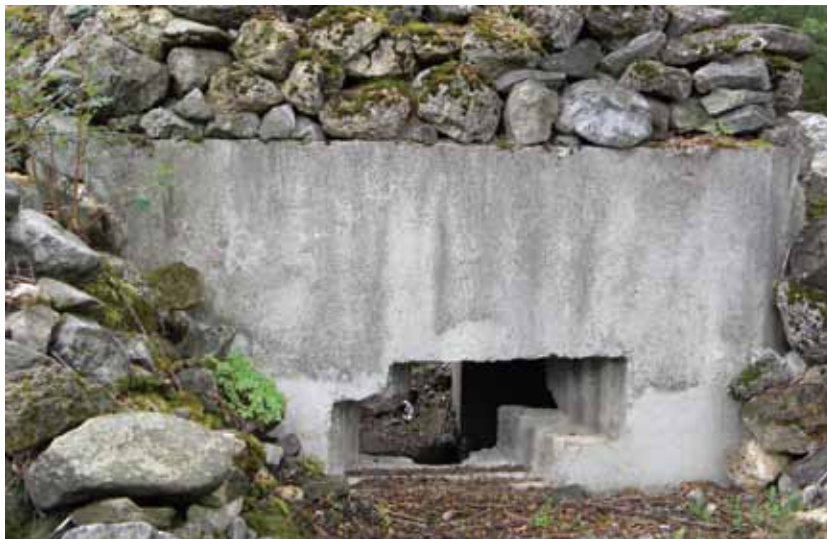
Figure 4: A French pillbox dating from 1939, probably for a 25mm anti-tank gun, at La Vachette close to the Italian border in the south east of the country. Associated with this work were shelters, infantry pillboxes and mine chambers forming a valley barrier and part of a network of defences along the border.
