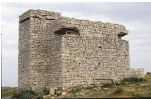
Figure 5: A British pillbox on Marfa Ridge, Malta, dating from 1935. It is carefully camouflaged with stone to resemble local buildings. The corner embrasures for machine guns are a characteristic of Maltese pillboxes. Note the observation position in the top of the ventilator.
