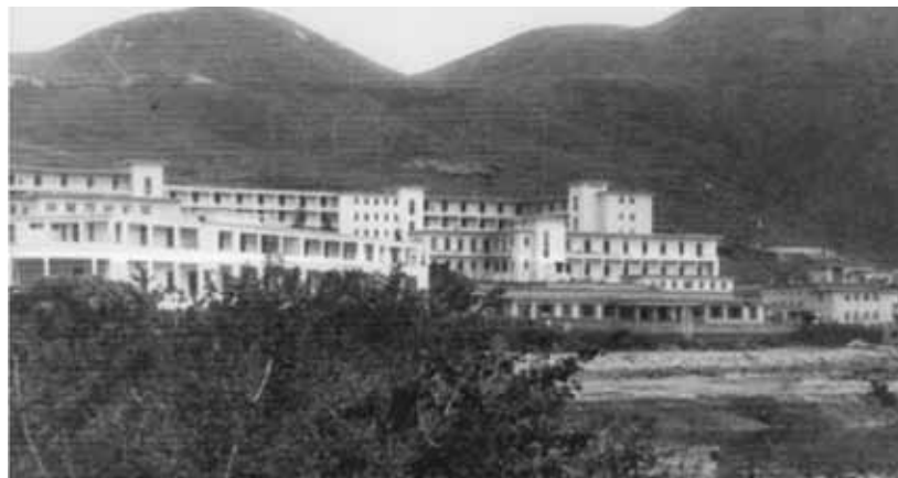
Figure 1: Little Sai Wan Complex
