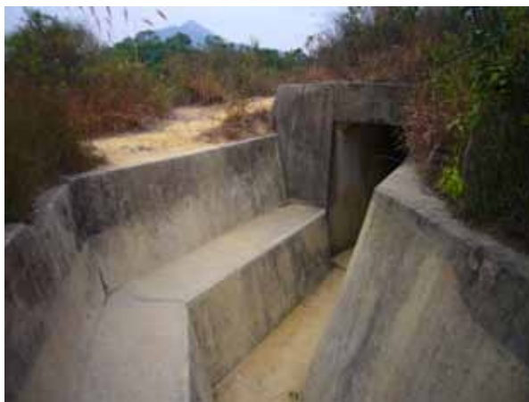
Figure 15: Trench near Strand Palace Hotel the kitchen of Shing Mun Redoubt Location E in Map 2. There are a number of similar open air trenches linking and in between the 'Underground' Tunnel System. These used for gun and mortar firing. This location is close to kitchen area and Charing Cross. [Editors' notes: T3, Figure 2, Lai, Ching, Davies and Wong (2011), this issue.]
