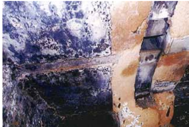
Figures 11a & 11b: The ventilation duct in the damaged wall. Note the vertical duct in the roof.
