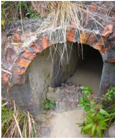
Figure 13b: Ruinous entry to the site of PB403, Shing Mun Redoubt Location F in Map 2. A number of tunnel entrances showed a brick vaulted lined construction method. This one connects to a PB403. Refer location F Map 2.
