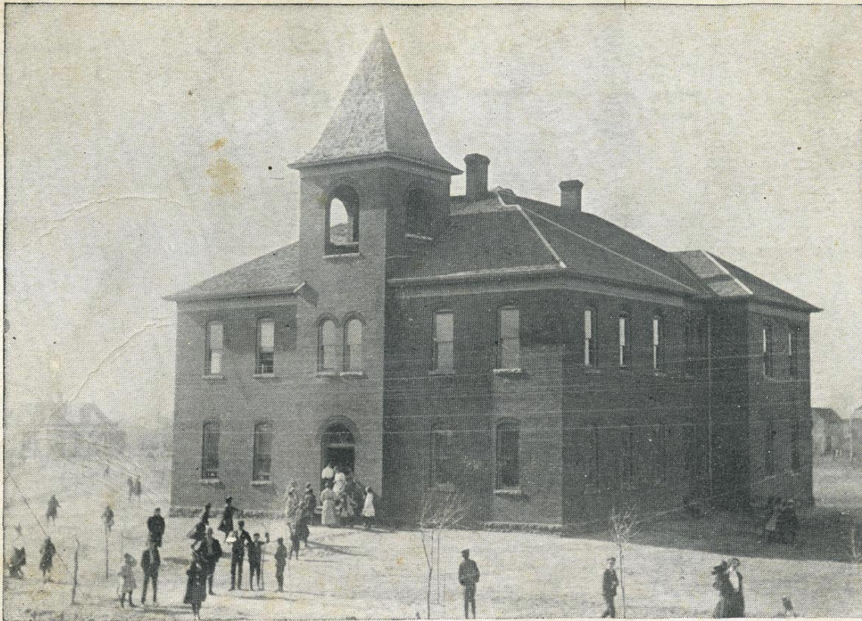
Watonga, Okla., High School Building.
