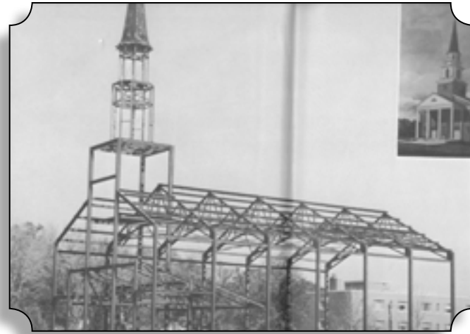
HARMAN CHAPEL CONSTRUCTION, 1965
