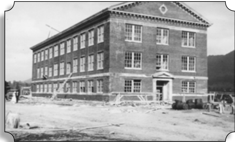
THE CONSTRUCTION OF LANSDELL HALL, 1922, BC'S FIRST BUILDING.
