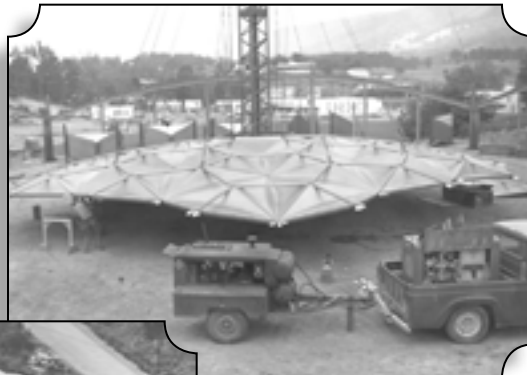
GOLDEN DOME CONSTRUCTION, 1968
