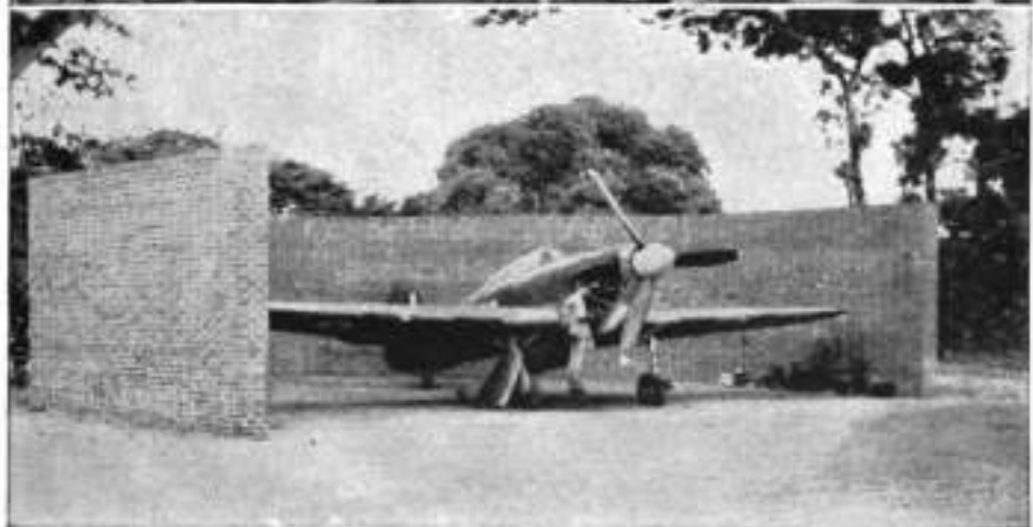
Old methods meet new, in construction of a brick dispersal pen to protect a parked Hurricane fighter from bomb fragments. [Tengah Airdrome, Singapore]
