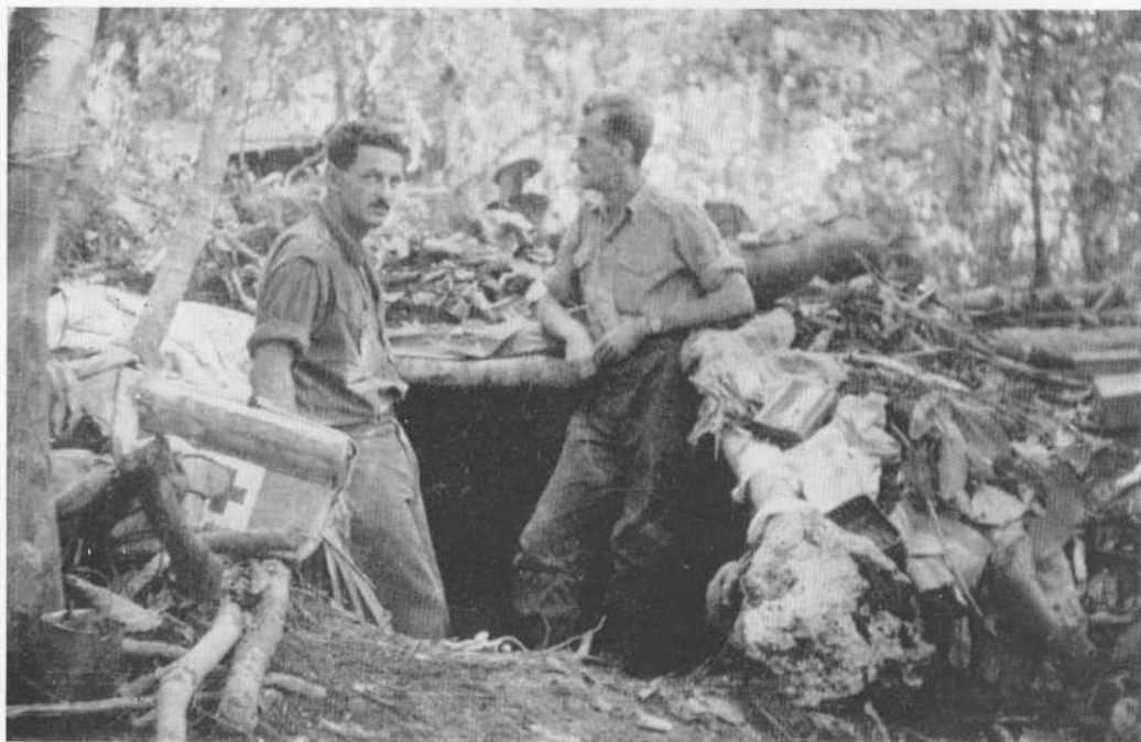
The R.A.P., 2/32nd Battalion at Pabu Ridge. It consisted of a shallow trench covered with timber and earth.
