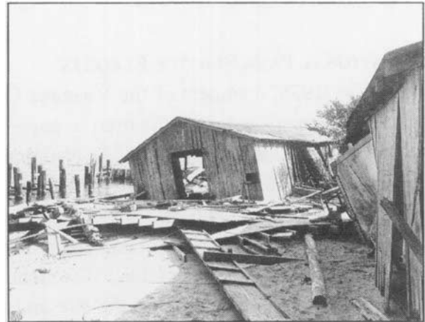
Figure 42. Damage to Waterside Theater caused by Hurricane Donna, October 14, 1960
