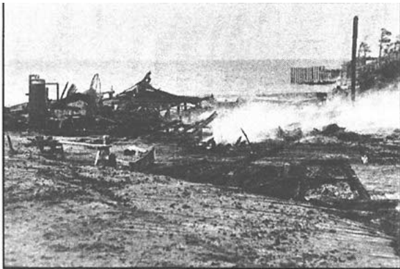
Figure 39. Waterside Theater fire damage, July 1947
