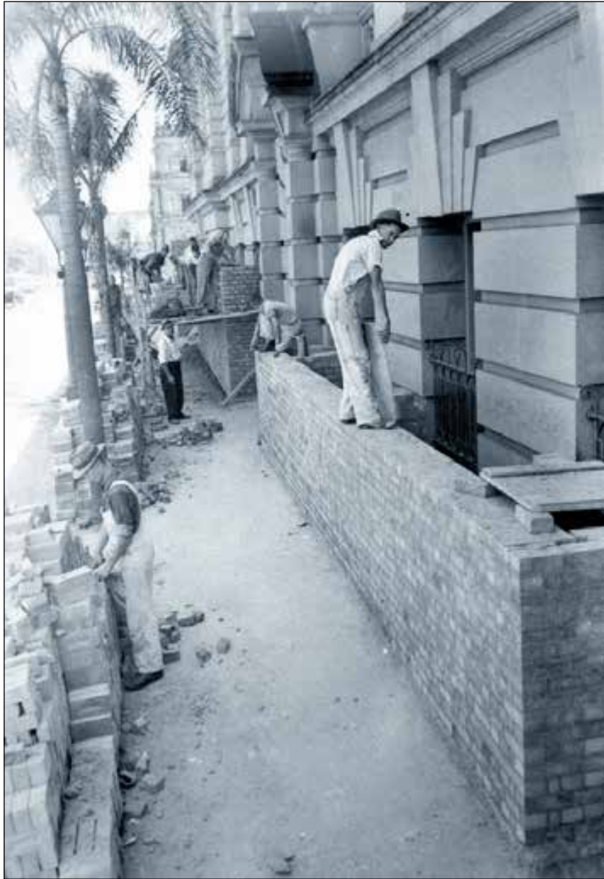
Workers prepare public buildings for air raids by removing plate glass windows and constructing brick screens, Brisbane, December 1941. (AWM 042765)
