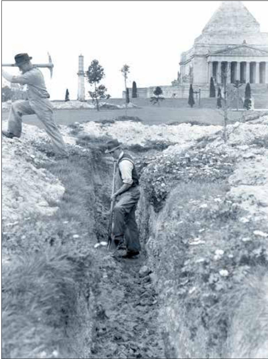
Men dig slit trenches in the lawns of the Shrine of Remembrance, Melbourne, in October 1942. (AWM 026959)
