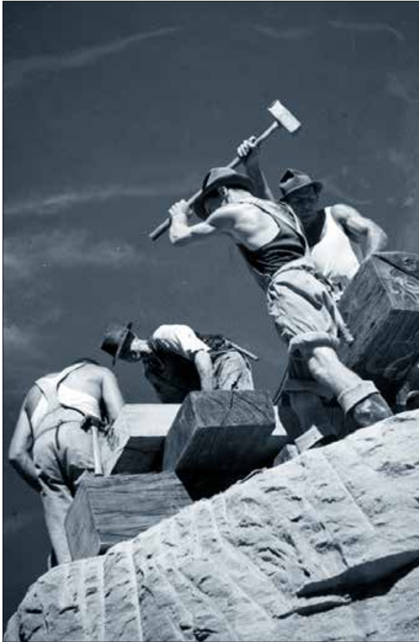
Members of the Civil Construction Corps work on an Allied Works Council project, c1943.
