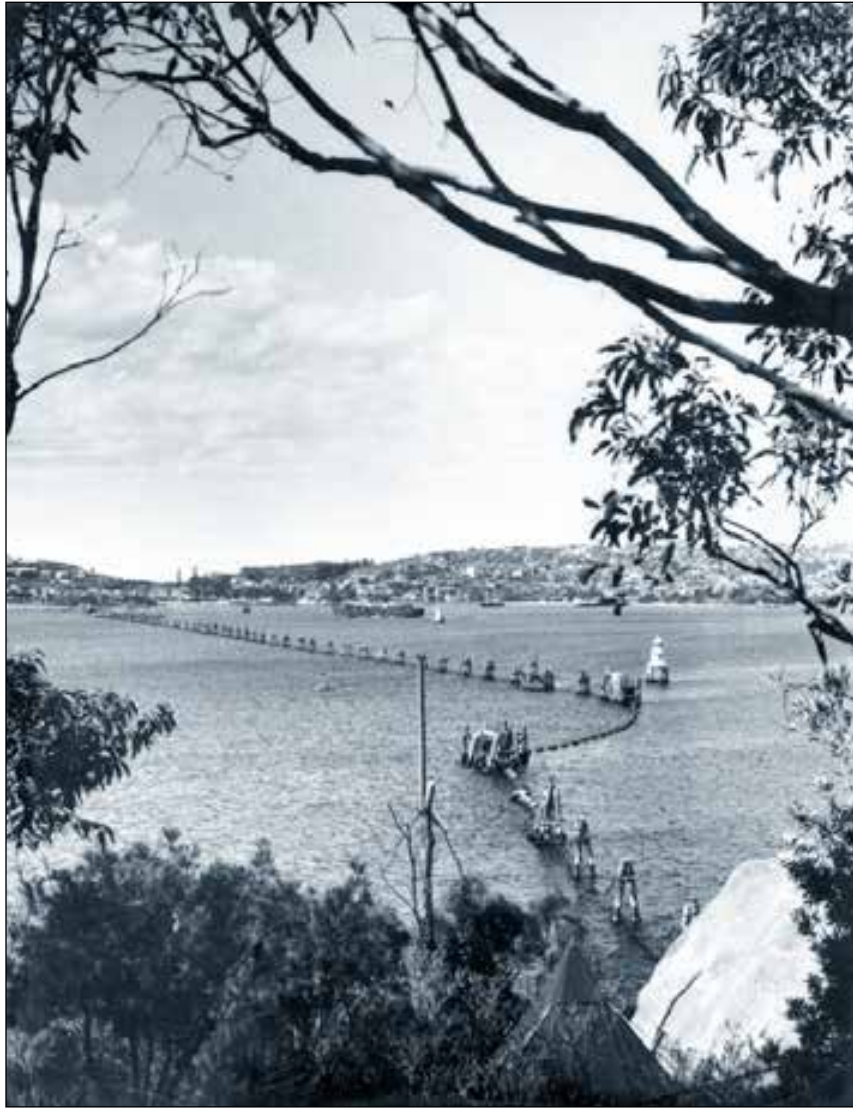
Sydney's boom defences, viewed from George's Head, c1942. At the time of the midget submarine raid only the centre section was complete. Construction of the single line steel anti-submarine net was begun in January 1942 at the narrowest point of the inner harbour entrance—between Green Point, on Inner South Head, and George's Head, on Middle Head. One of the midget submarines became tangled in the centre section on the night of 31 May 1942 and was destroyed by the crew. (AWM P03338.005)
