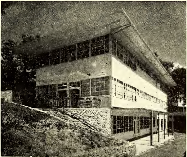
Center Building Constructed 1950-51, houses Nibble Nook, Baptist Book Store, barber shop, beauty parlor, and office of Relief and Annuity Board
