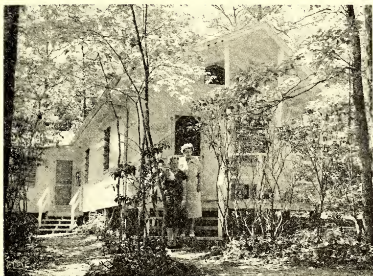
Administration Building, Camp Crestridge
