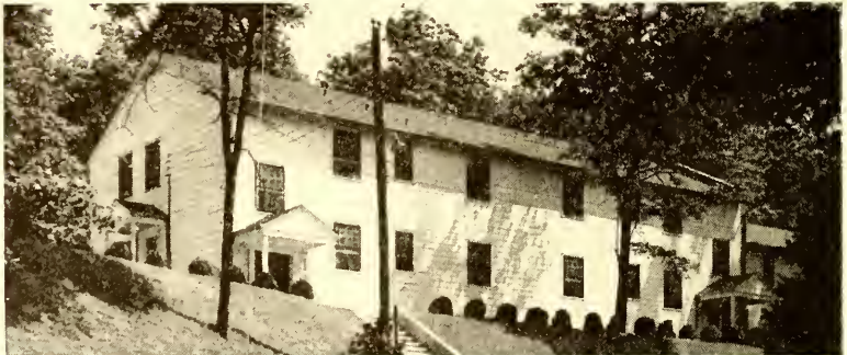
Springdale Annex Constructed 1925-26 as a cafeteria building, later remodeled into bedrooms; new wing of bedrooms with private baths added in 1949
