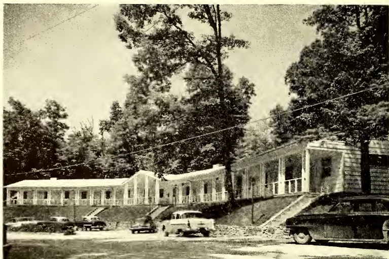
Florida Cove Apartments Constructed in 1955 with eight efficiency apartments accommodating six people each
