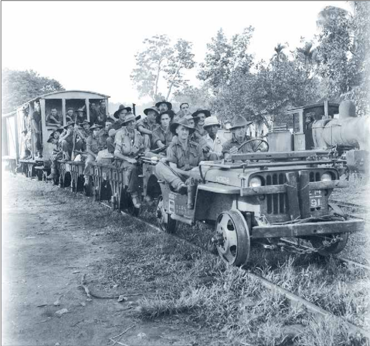
The celebrated 'Jeep Train', known as the Membukut Special, on the Beaufort-Jesselton railway. Engineers of the 9th Division repaired the railway, adapted jeeps to replace damaged locomotives and returned the railway to working order. (AWM 111845)
