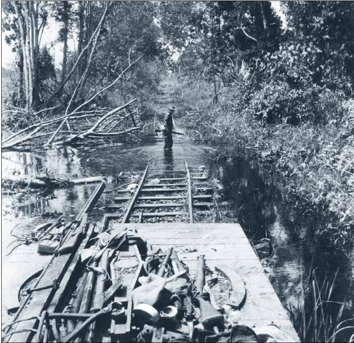
A soldier checks the condition of a section of the Beaufort-Jesselton railway line flooded by rains, ahead of the Jeep train crossing the swollen creek. Armed guards accompanied the train, and patrolled ahead whenever necessary, in case of Japanese parties infiltrating the Australian lines to attack the railway. (From the collection of Warrant Officer RH Campbell, HQ 24th Brigade)
