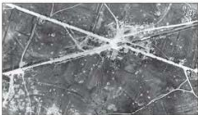
Aerial view of the town of Zonnebeke, 7 June 1917, before a major action. AWM J00188
