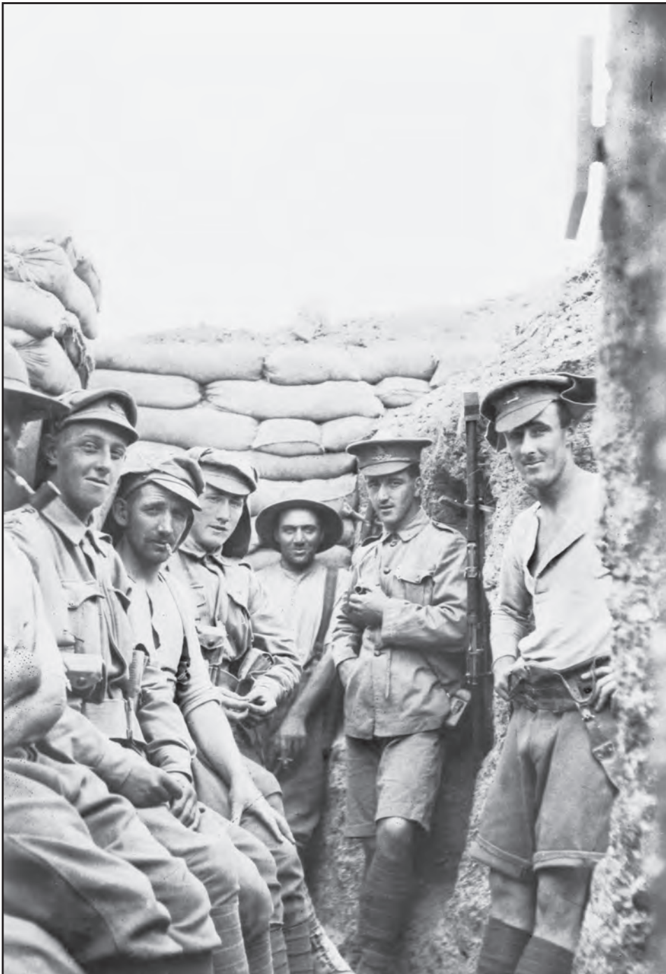
Image 1: A freshly dug trench
