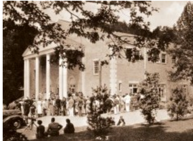
Spilman Auditorium Dedication, 1938
