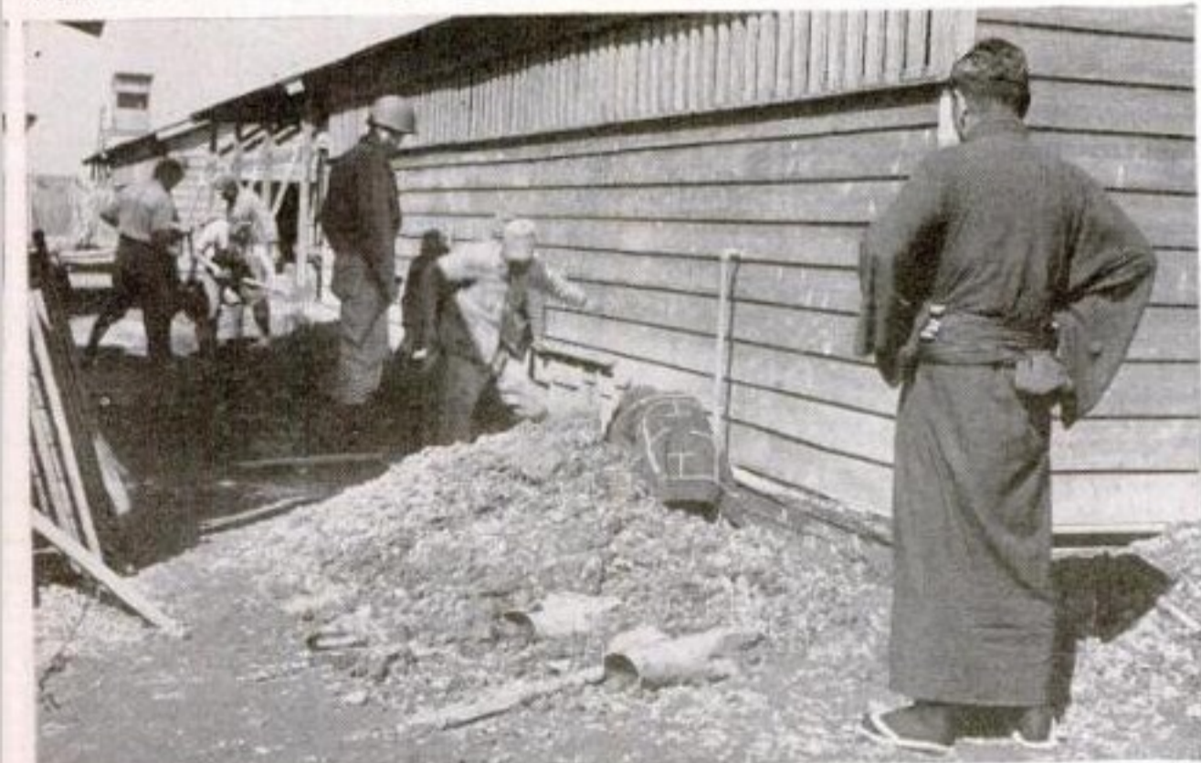
Sewage system, installed so that Omori camp will be in accord with the Geneva Convention, replaces the virtually nonexistent facilities provided U. S. prisoners at Omori. Here Minister Kishi looks on amazed. Jap soldiers do the manual work while the Americans direct them.
