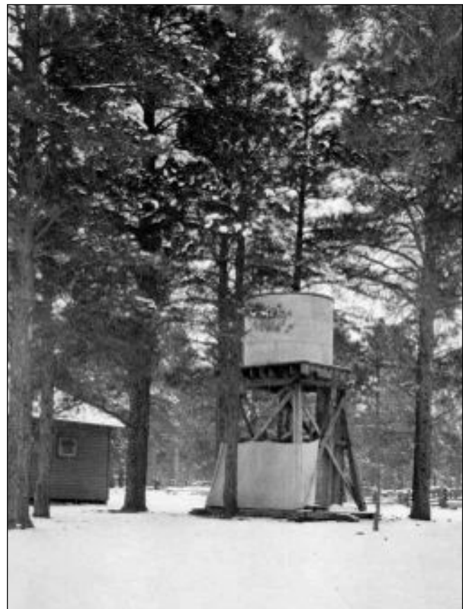
Figure 4. The water tank and bath house at FVEF. The mess house is to the left. USFS photo 92583 by G. A. Pearson in 1911.
