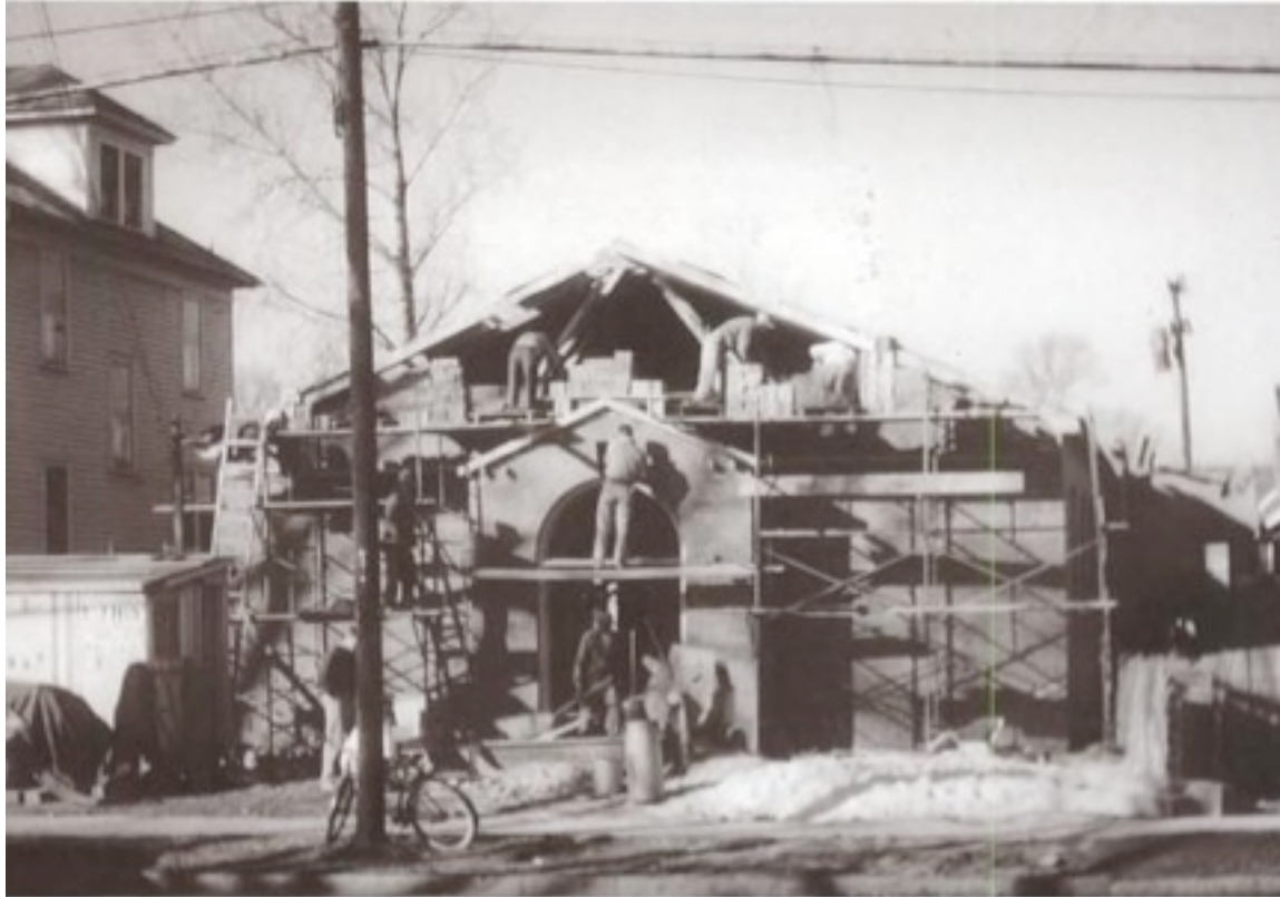
Chesapeake Avenue Methodist Church: Fellowship Hall, under construction, late 1950s (Baptist parsonage on left)
