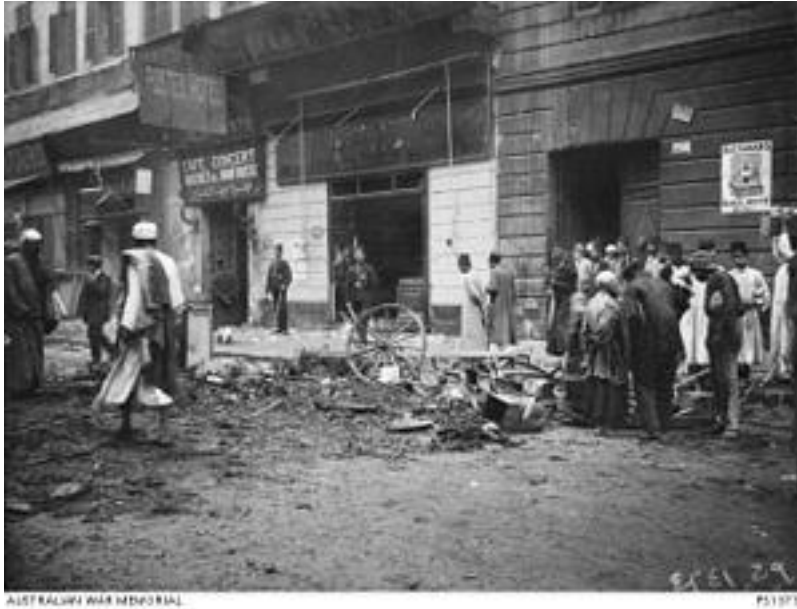
Damaged buildings in Cairo, possibly the aftermath of the riot
